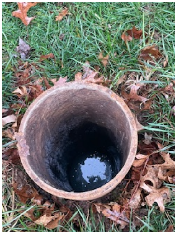
8" access into septic tank/cesspool
