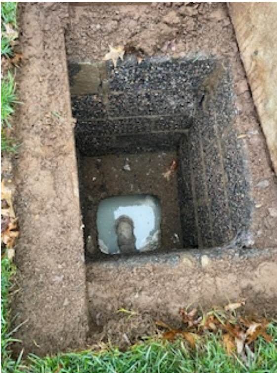
4" plastic elbow outlet baffle
