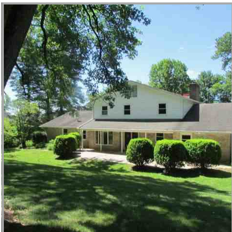
rear (from yard)
