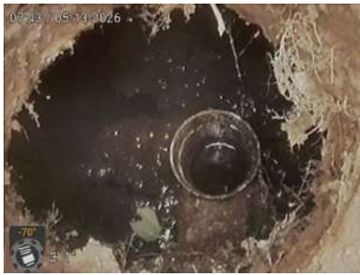
Inside the back of the septic tank
