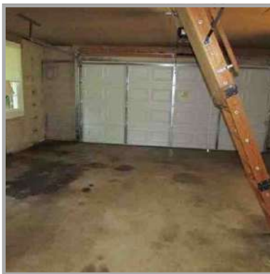
interior garage/attic entry
