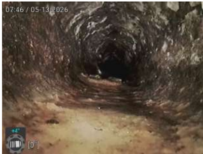
Inside cast iron sewer line from the tank towards the house
