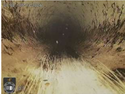
Inside PVC outlet pipe from tank to the distribution box
