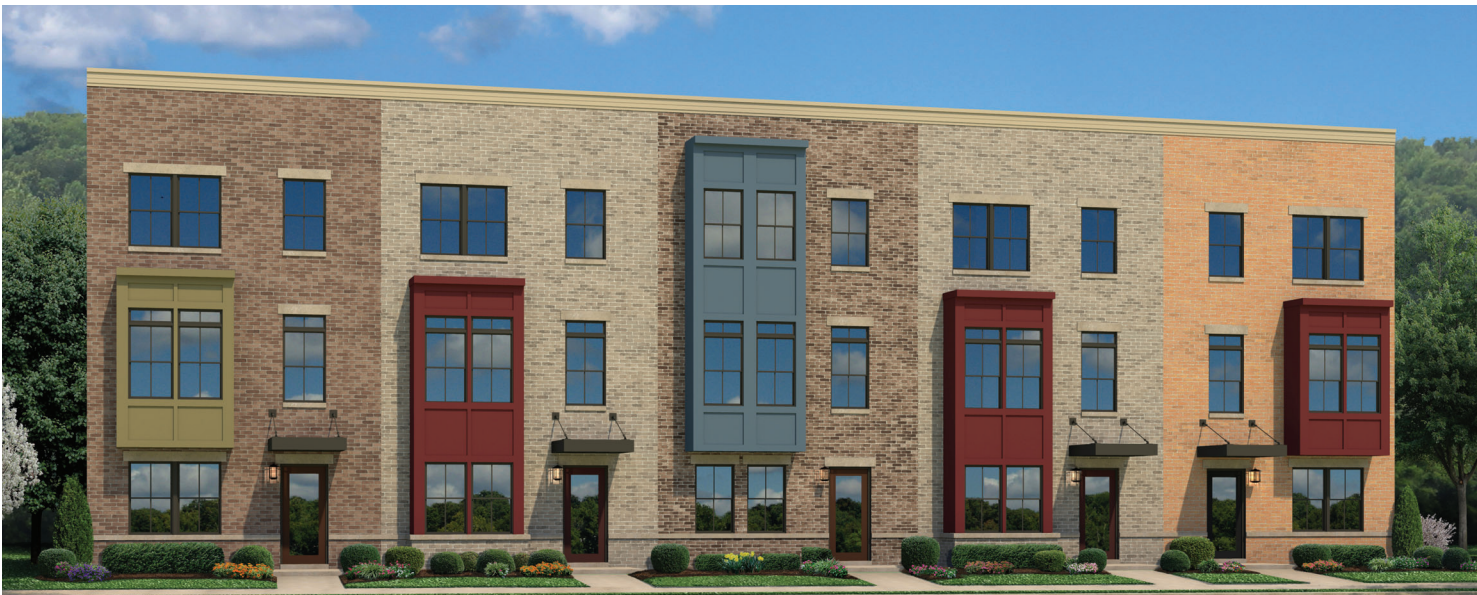
LOWER LEVEL ENTRY WITH REAR GARAGE
